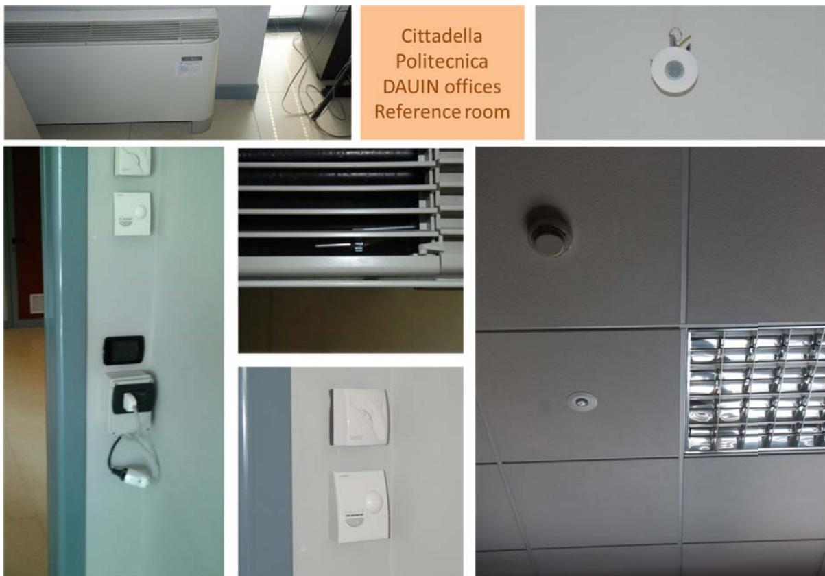
Figure 6: Wired sensors installed in the Cittadella Politecnica, DAUIN Offices, Reference room.
