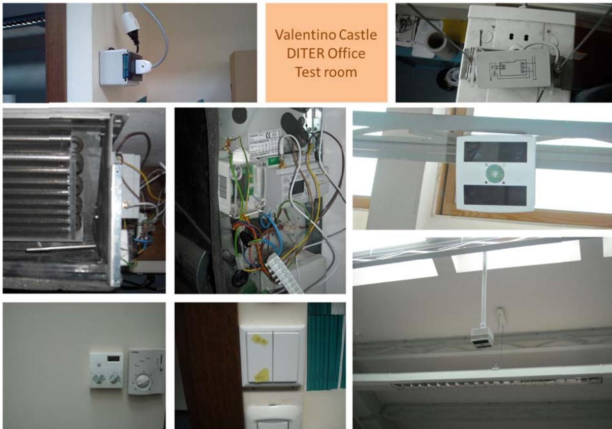
Figure 9: Wireless sensors installed in the Valentino Castle, DITER Offices, Test room.
