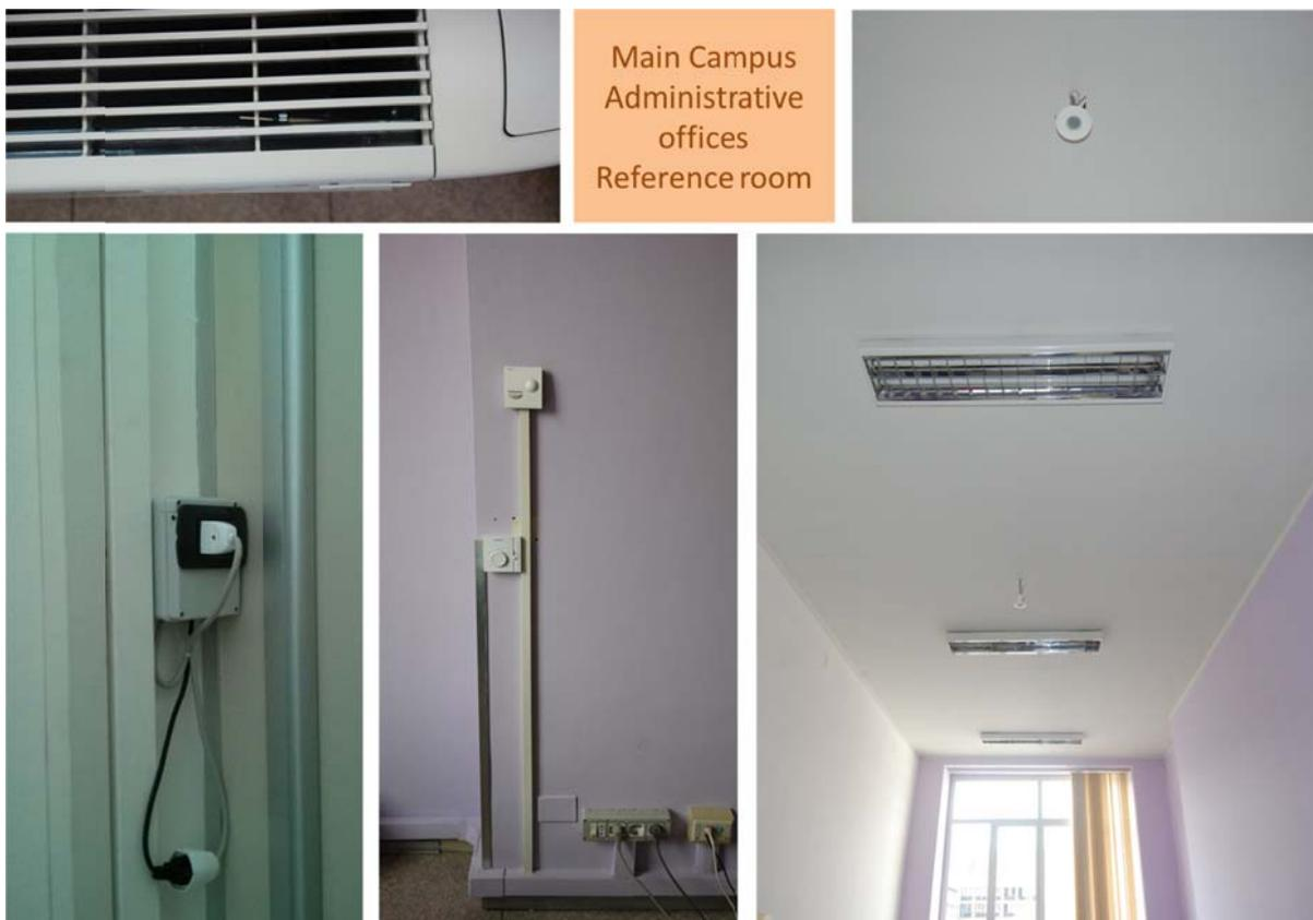
Figure 8: Wired sensors installed in the Main Campus, Administrative Offices, Reference room.
