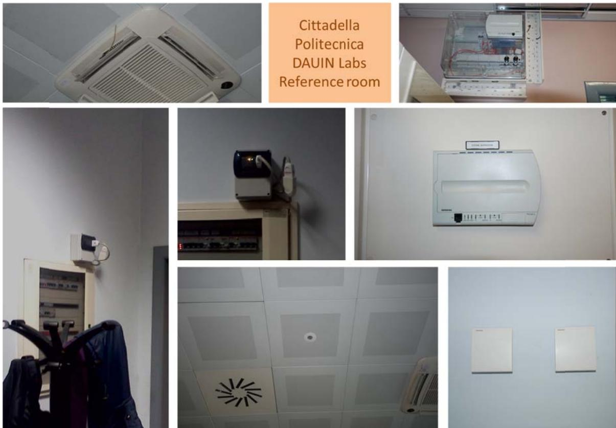
**Figure 4: Wired sensors installed in the Cittadella Politecnica, DAUIN Labs, Reference room.**
