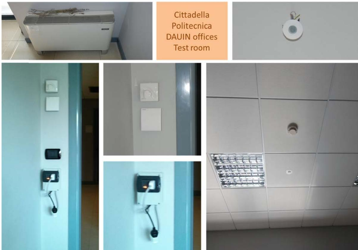
Figure 5: Wired sensors installed in the Cittadella Politecnica, DAUIN Offices, Test room.
