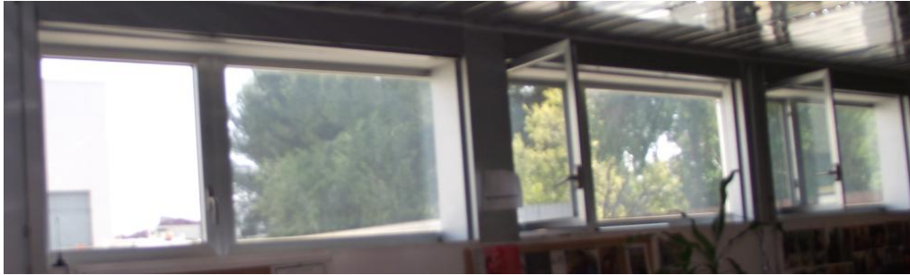
Image of PICA building First Floor Façade Window Opening
