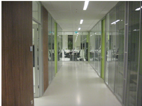
Internal Views of HHS – Indicating Knoholem Project Areas fully glazed Corridor partitions
