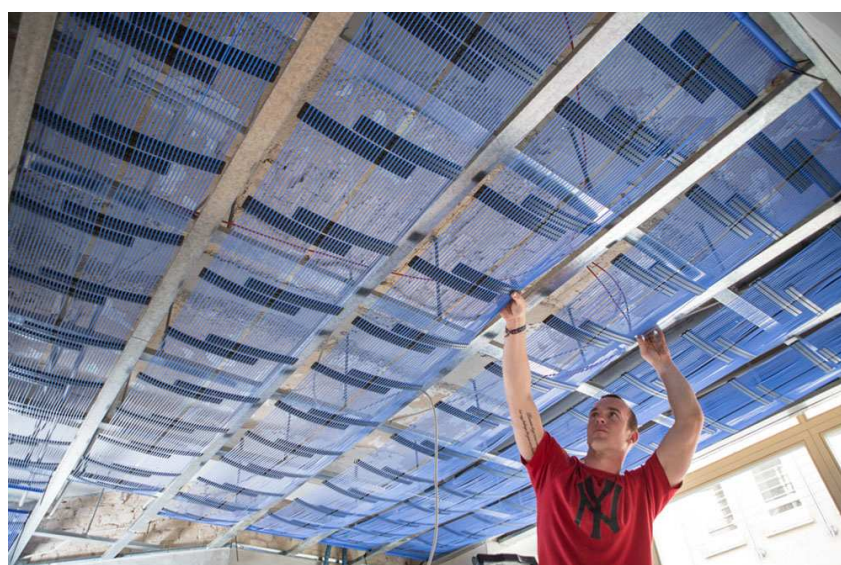
Figure 1 Installation of Capillary tube system
