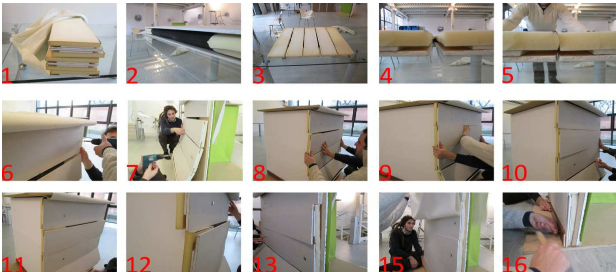
Fig. 18: Sequence of assembly.
