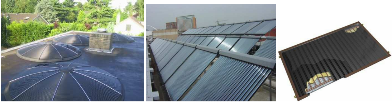
Figure 23. Swimming pool collector (sundisc), Evacuated tube collector (Soltech Int. Co), Flat plate collector (21st century solar).
