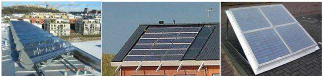
Figure 51. PVT collectors (a) Concentrating collector, (b) Unglazed PVT air collector, (c) glazed PVT liquid collector.
