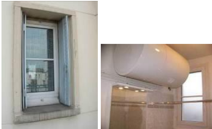
Figure 2 and 3. PVC windows with metal blinds (before renovation) and individual electric boilers in bathrooms (before renovation)
