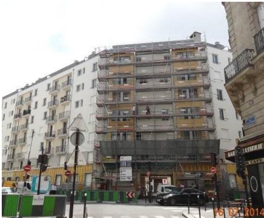
Figure 6 The Paris building during retrofit (source: ICF Novédis)
