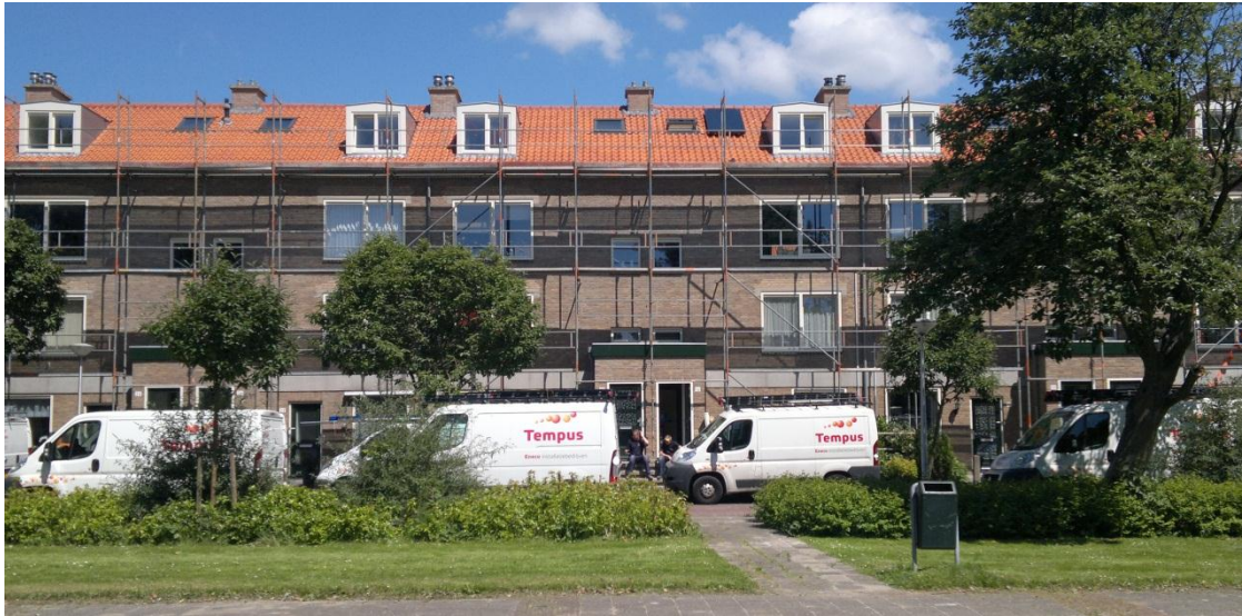
Figure 7 The Delft buildings during installation of solar panels (source: Woonbron)
