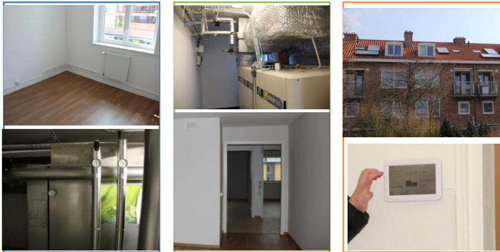
Figure 5 Building services after retrofit: Examples from the HVAC, DHW and ICT systems after retrofit for (from left to right) Paris, Alingsås and Delft. Tenants were also encouraged to switch to low energy lighting.
