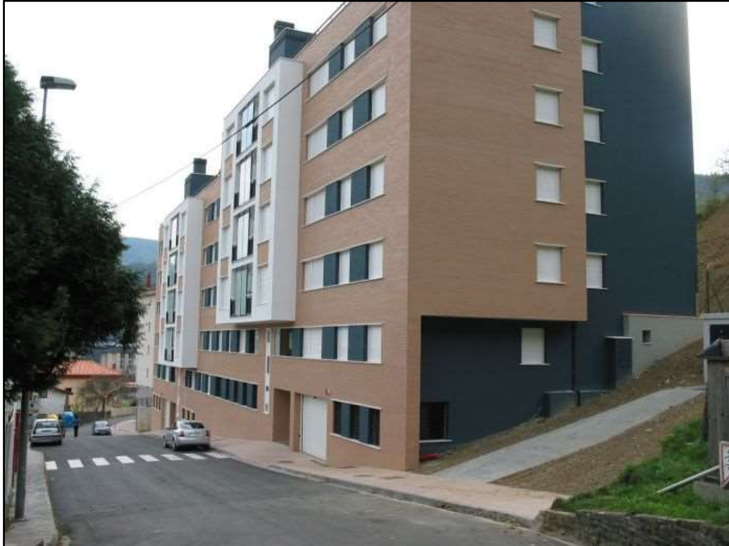
Figure 59 - Building general view (2)
