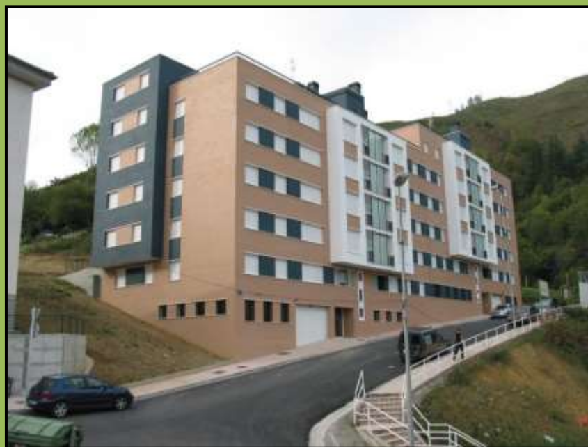
Figure 1 - Building general view
