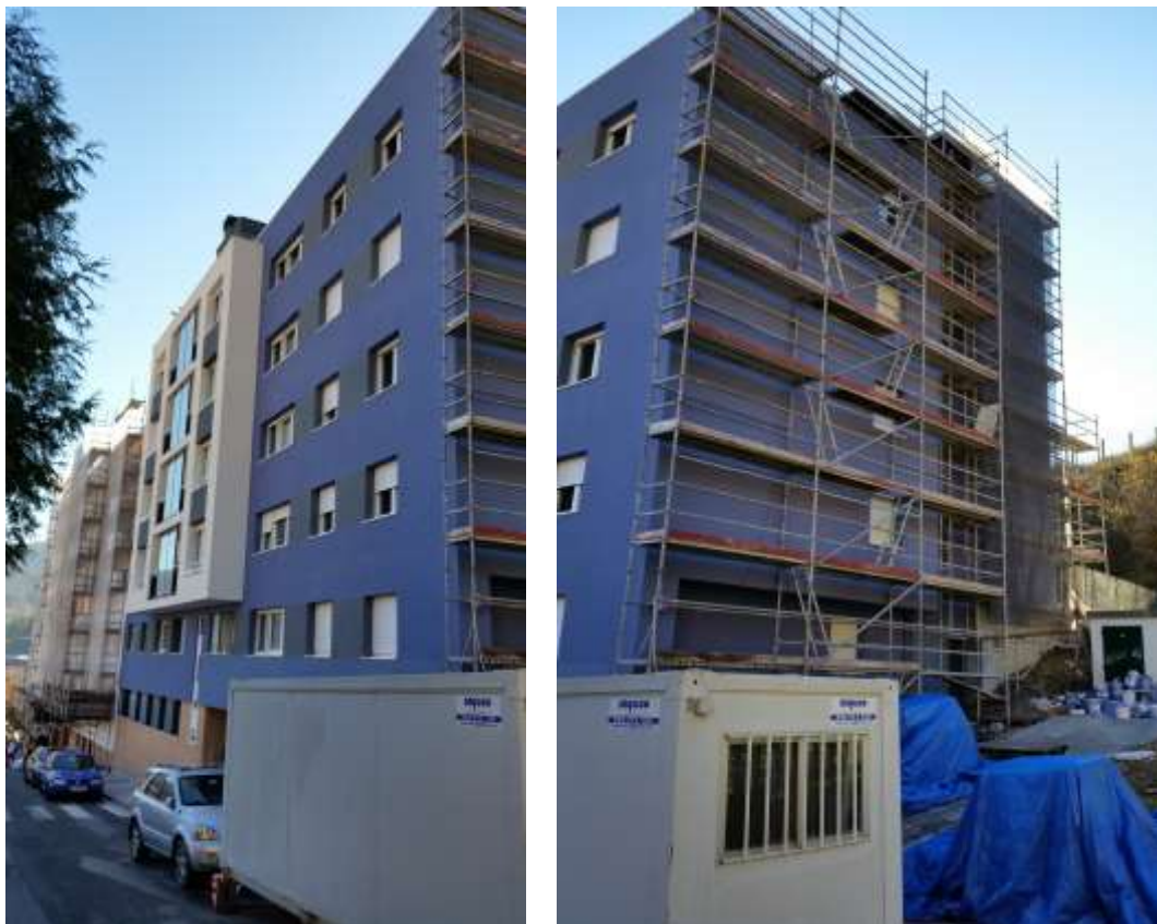
Figure 67 - Scaffoldings during the work.
