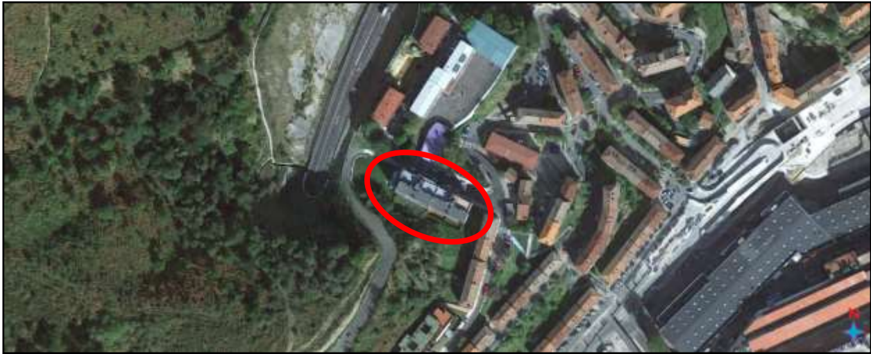
Figure 57 - Building aerial view.
