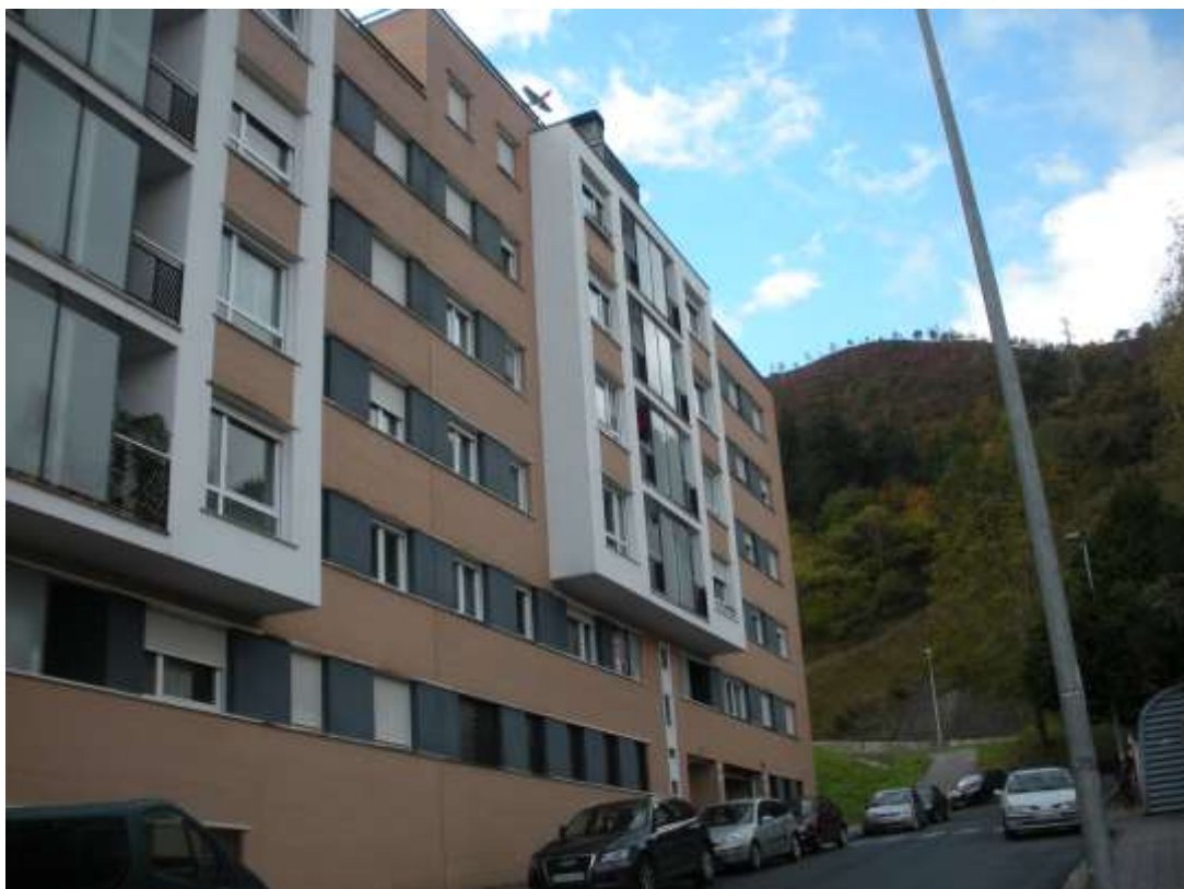
Figure 60 - Building general view (3)
